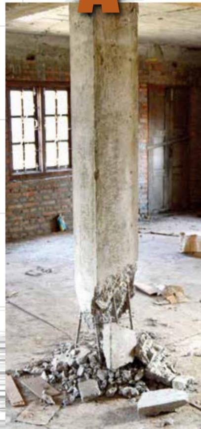
The Purdue team documented damage such as this case of combined shear and axial (compressive) failure of a column.
