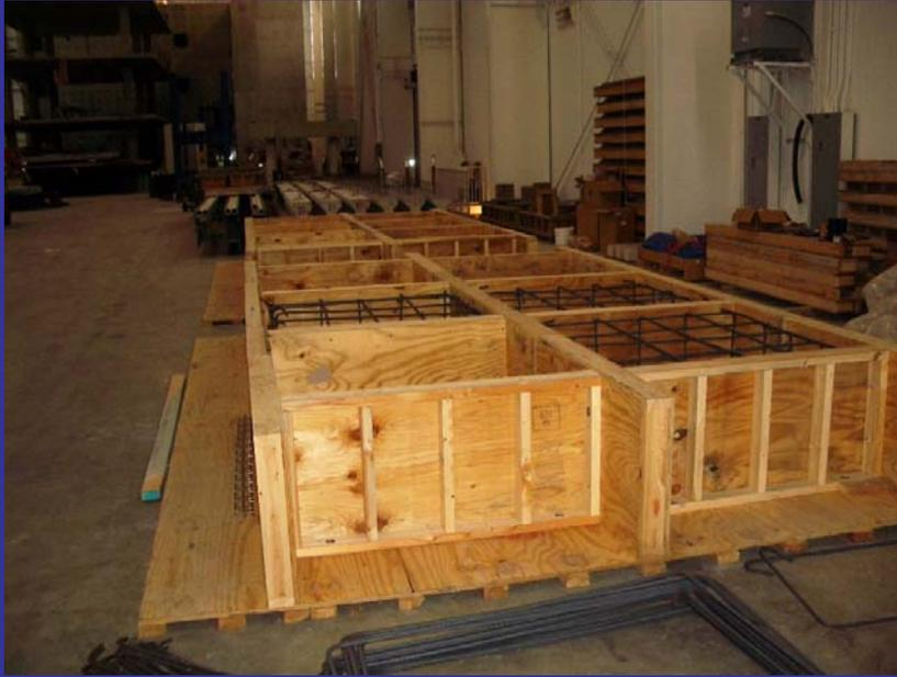
**Formwork and Reinforcement Before Casting of Support Blocks**
